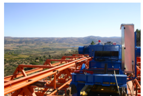
Detail of the winch used to open and close the formwork panels
