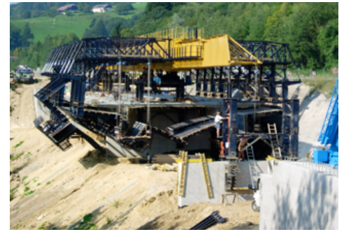
Formwork opening
