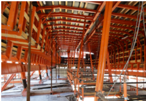
Internal formwork
