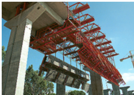
Formwork panels at open position during launching
