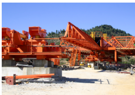
Temporary support behind the abutment
