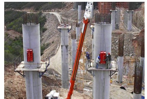
Installing steel brackets at short columns to support transverse steel beams
