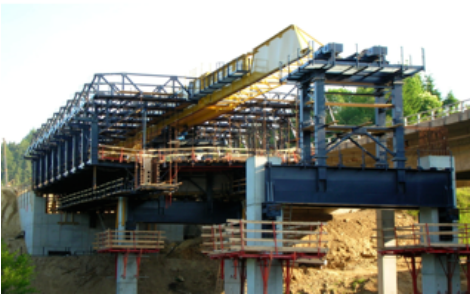
Supports installed on top of transverse steel beams anchored to the columns
