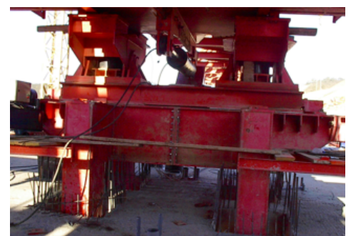
Upper part of the main support and launching wagon used at launching and side shift
