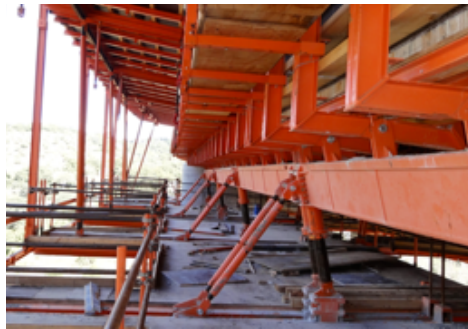
External formwork
