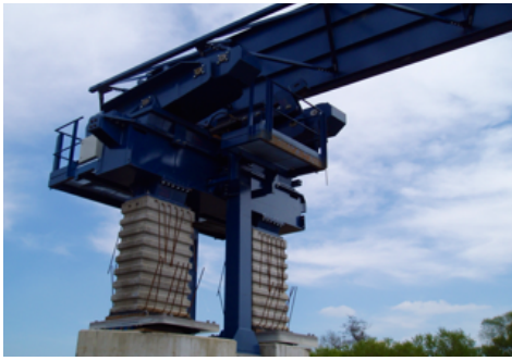
Special front support using concrete prefab legs.
