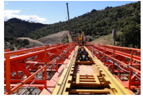
Rail and winch used to open and close formwork panels
