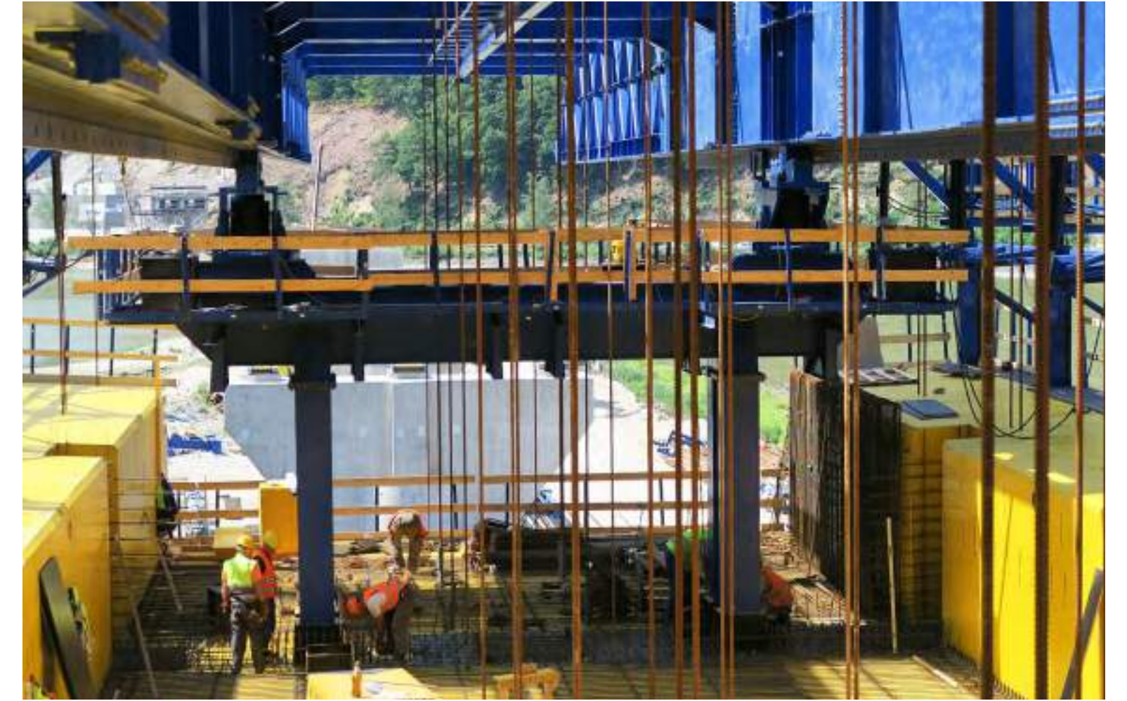
Overhead MSS front support – Bystrica, Slovakia
