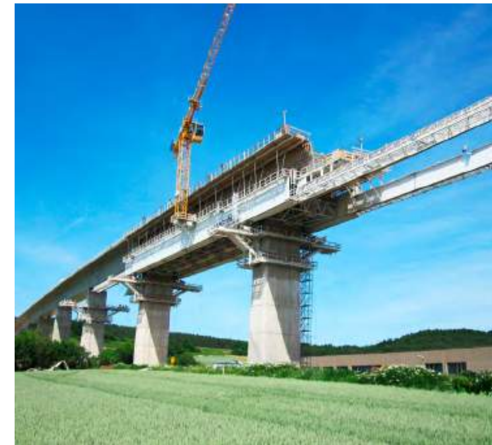
Underslung MSS – Füllbachtal, Germany
