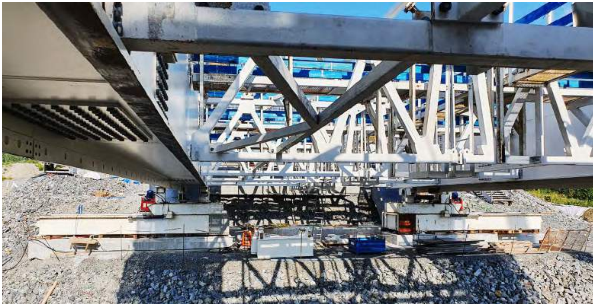
Temporary support close to abutment – Randselva, Norway
