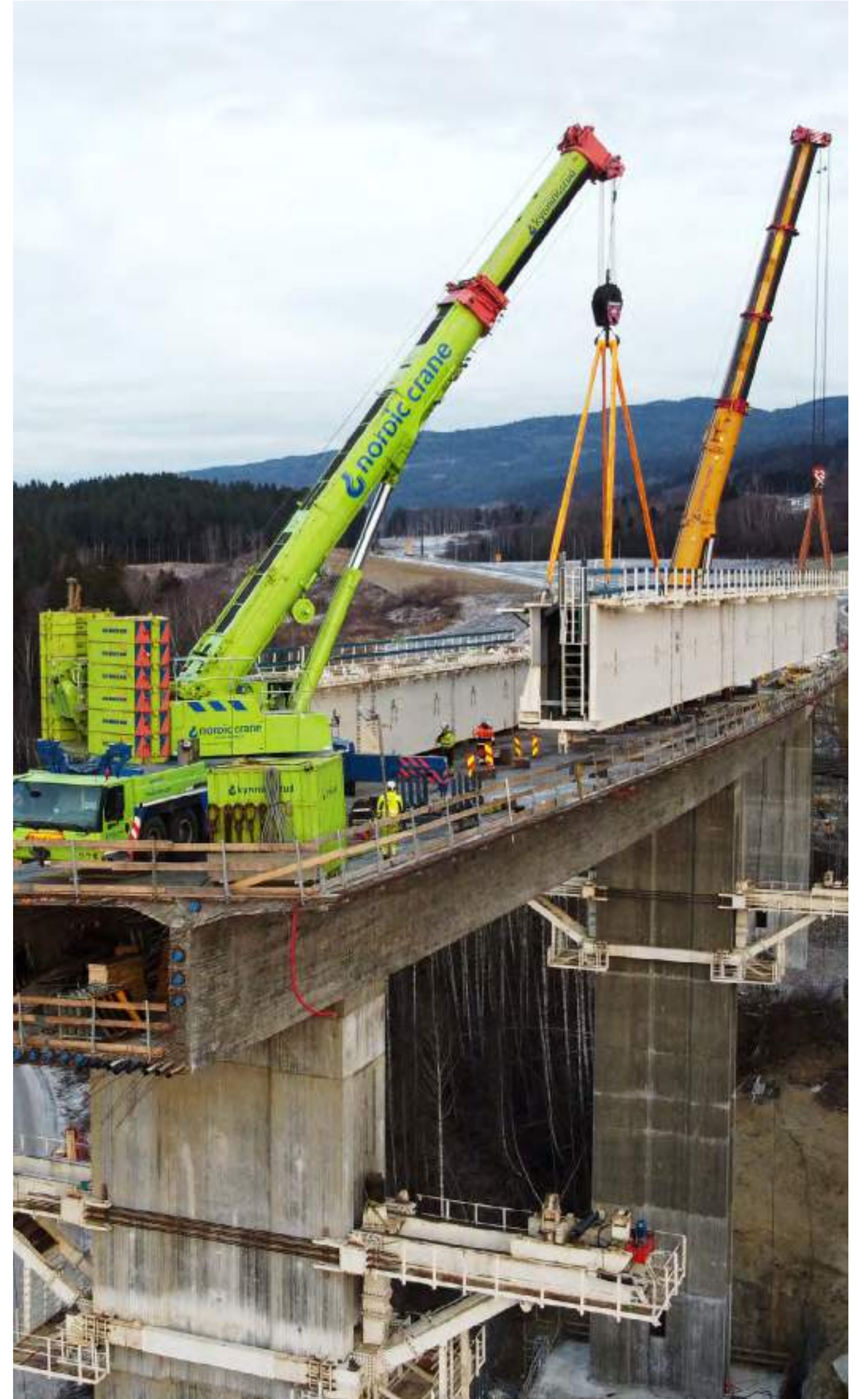
MSS dismantling – Randselva, Norway
