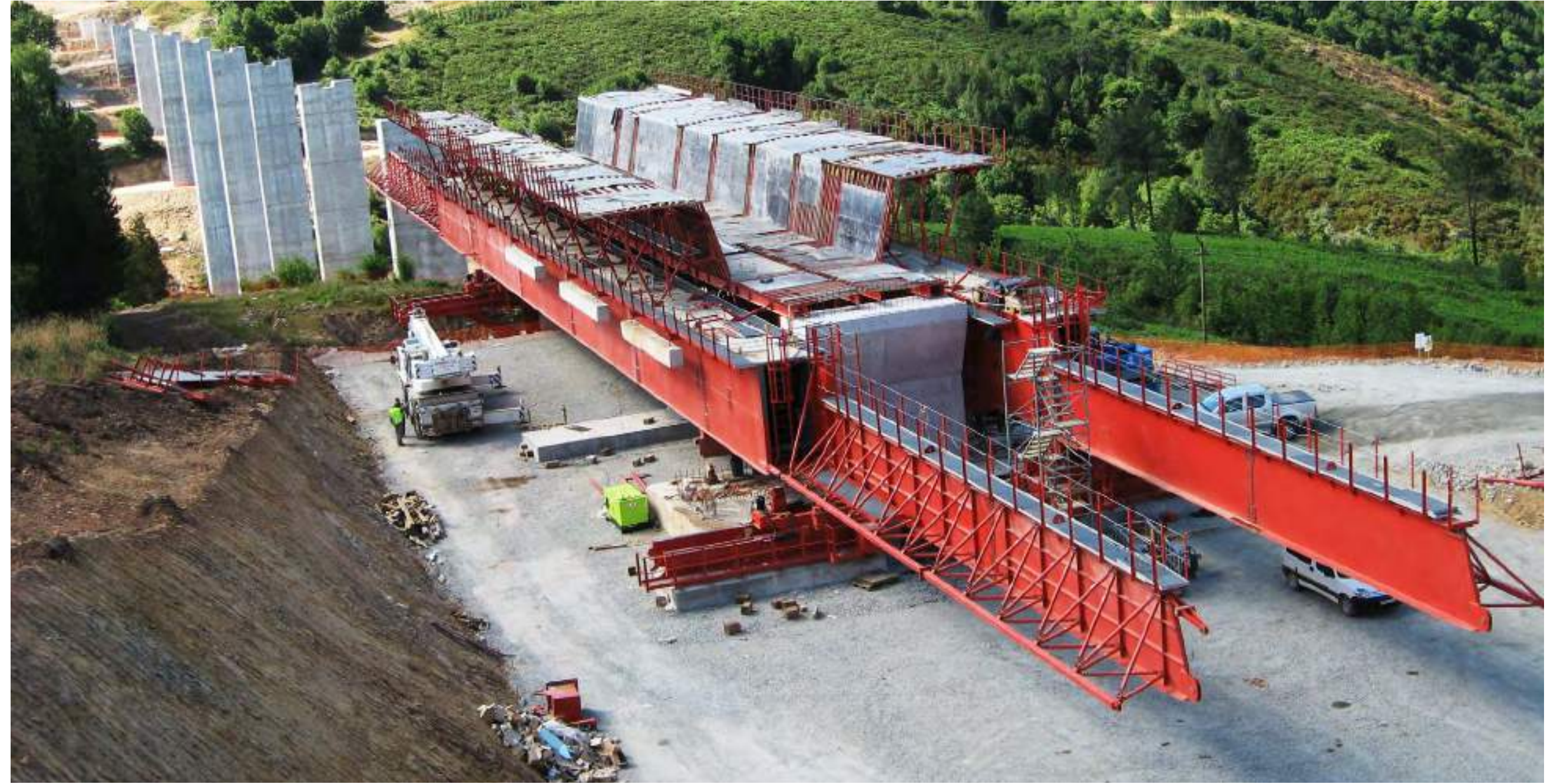
Underslung MSS – Cabirtas, Spain
