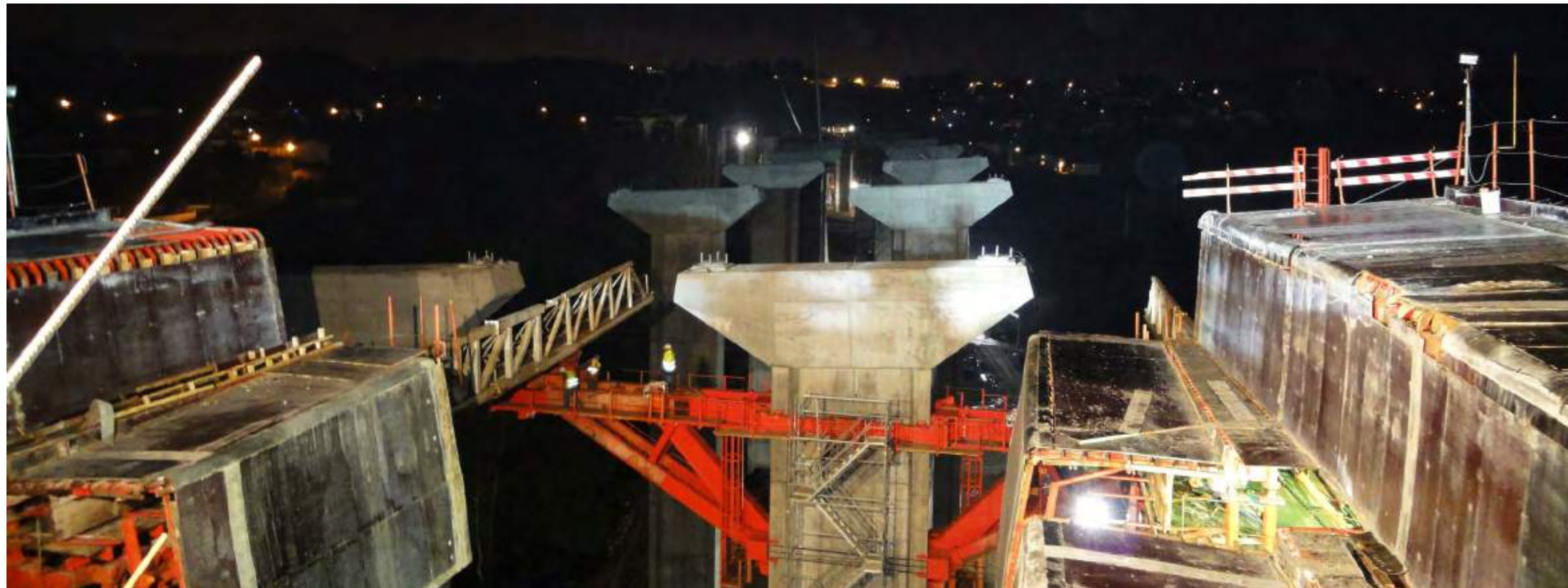
Internal formwork in the open position
