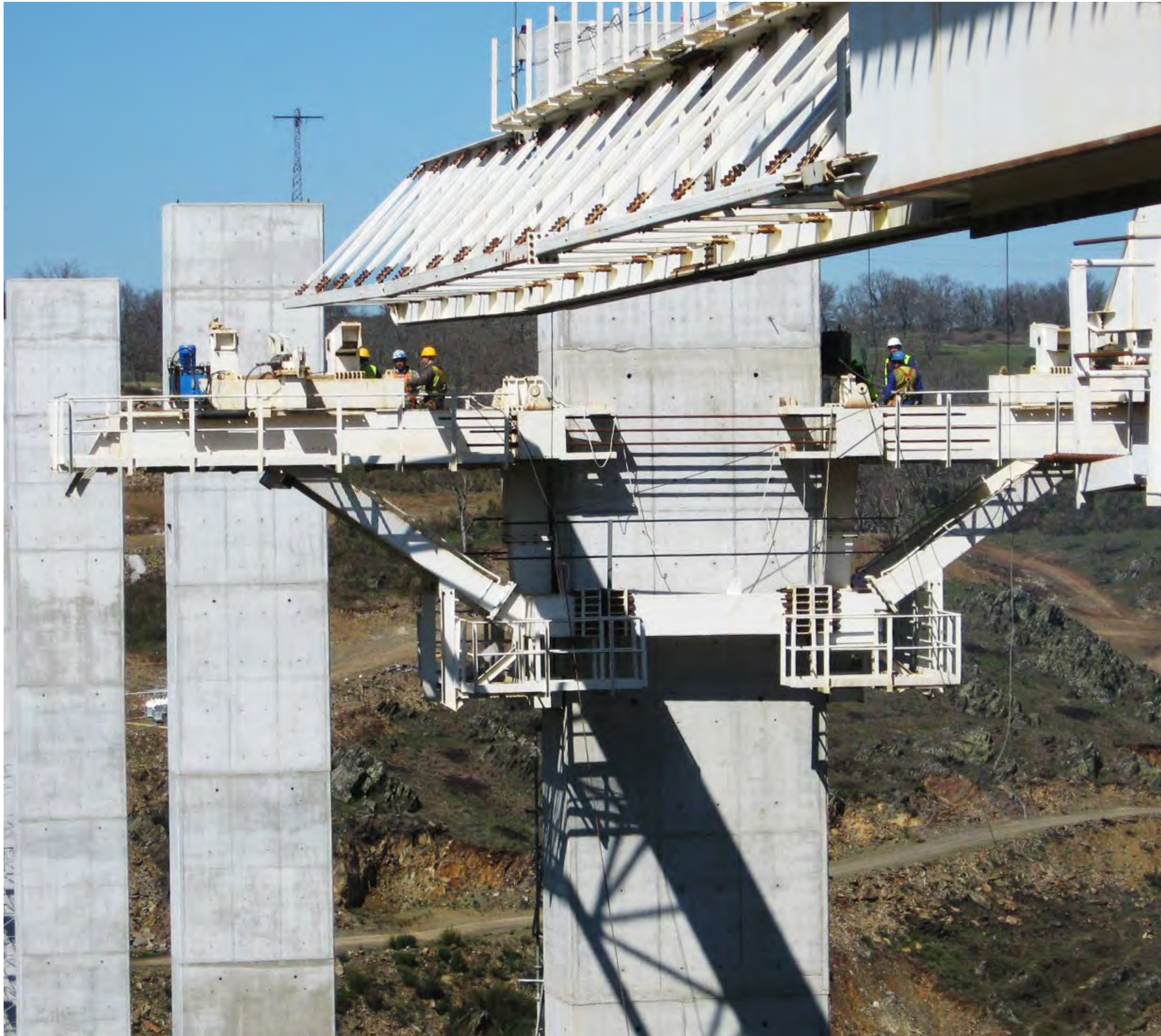
MSS launching– Salamanca, Spain
