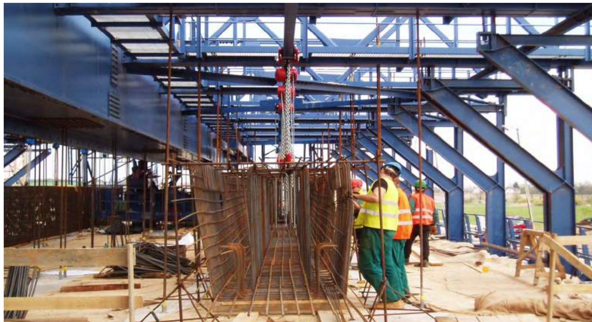
Overhead MSS – transporting the rebar cage using winches
