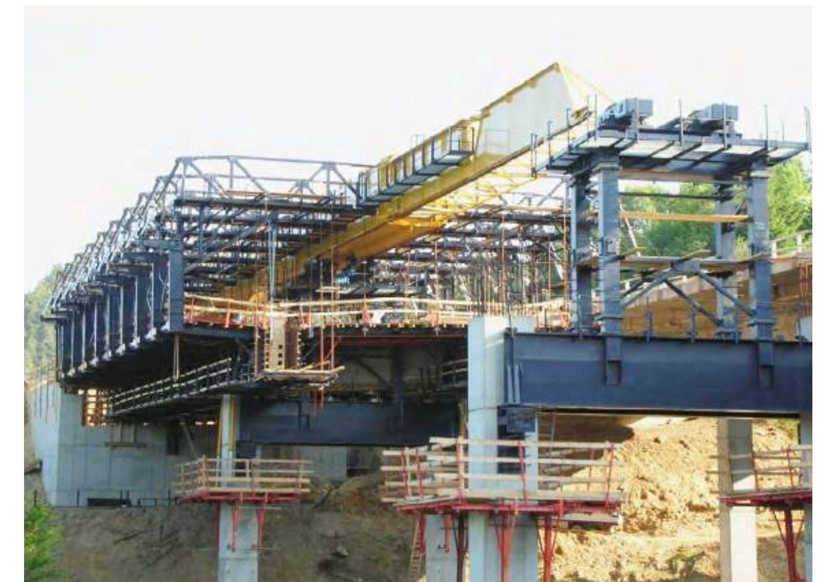
Crossbeam supported on the columns
