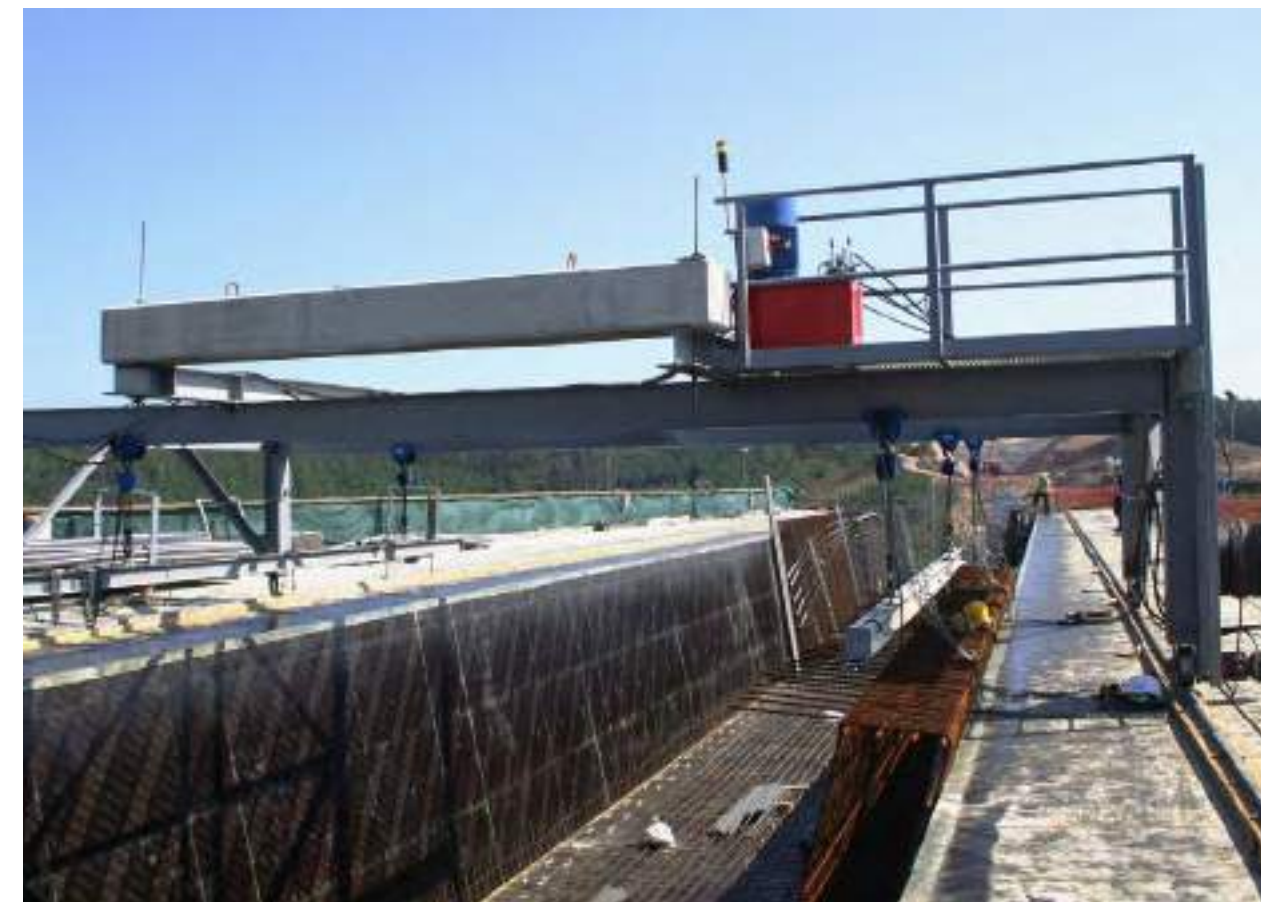
Underslung MSS – transporting the rebar panels using a transport trolley
