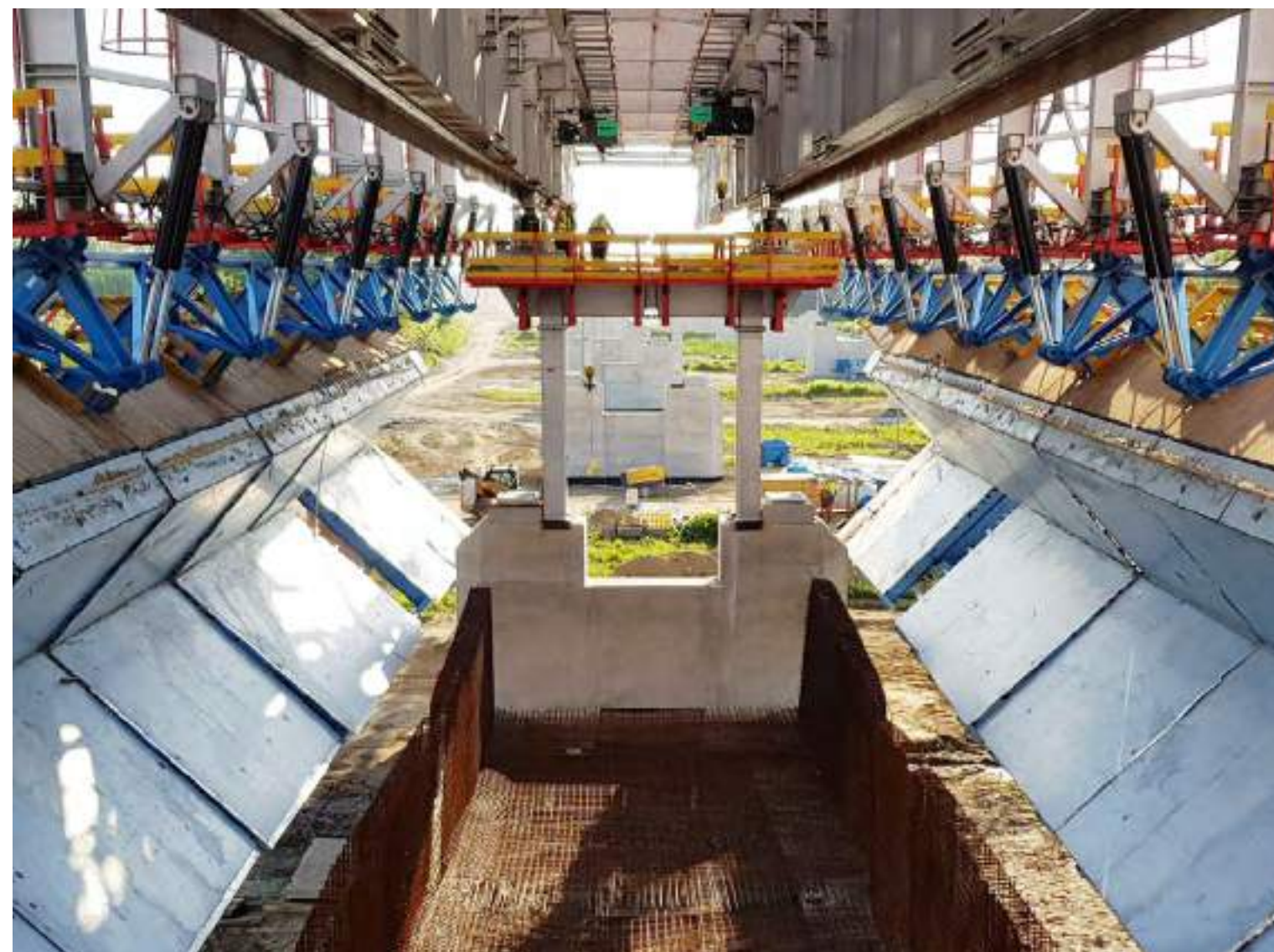
Direct support on the column
