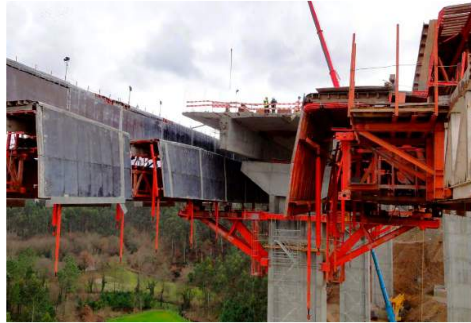
Internal formwork in the open position
