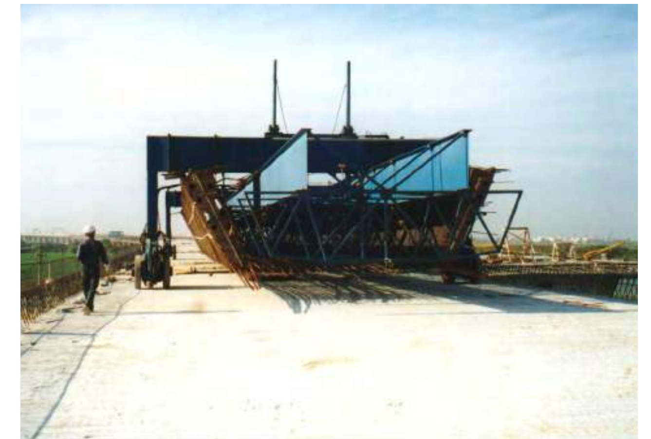
Underslung MSS – transporting the full span rebar cage
