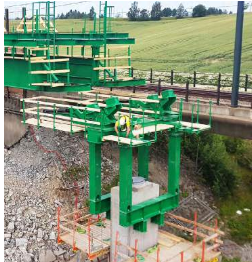
Profiles passing through the column
