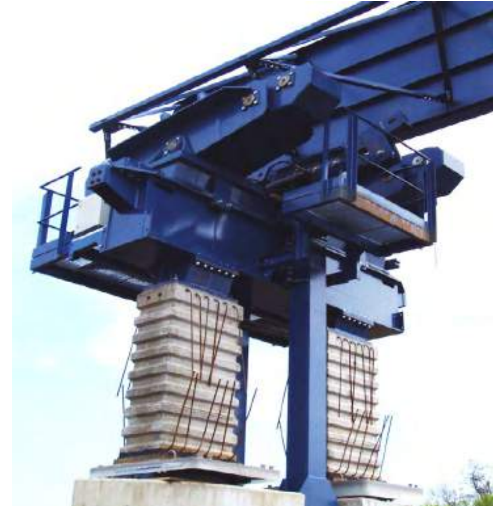
Concrete legs support
