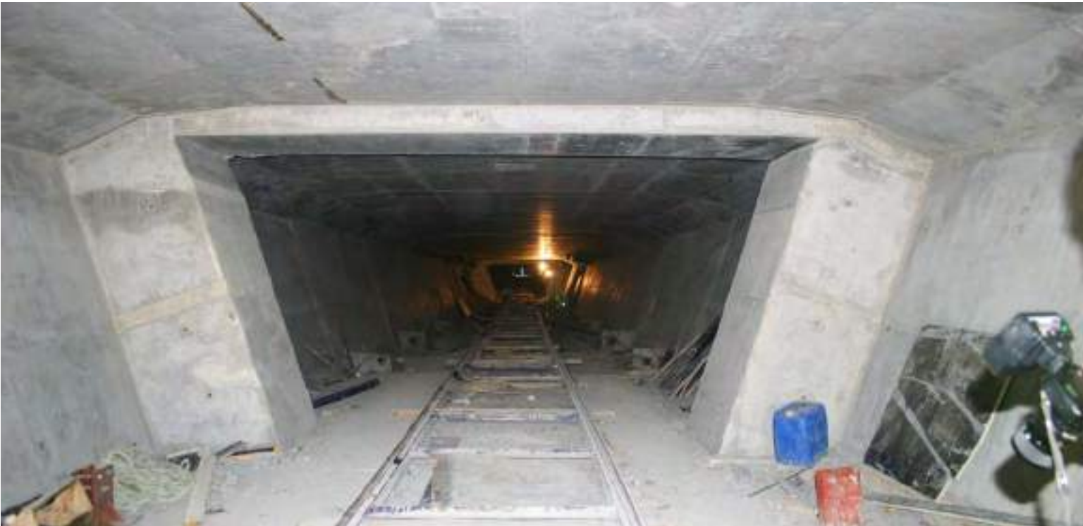
Column section deck diaphragm
