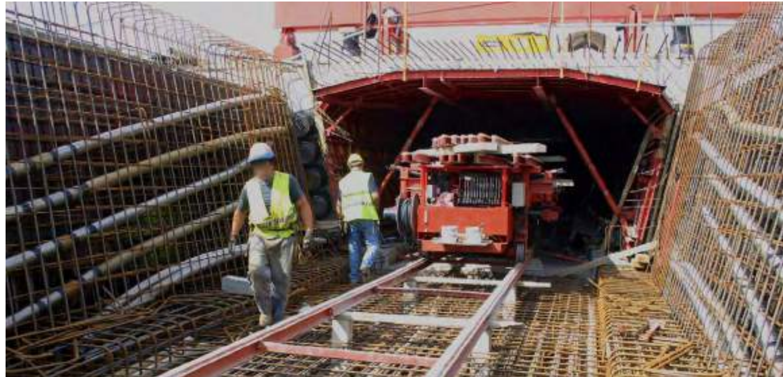
Formwork panel transport
