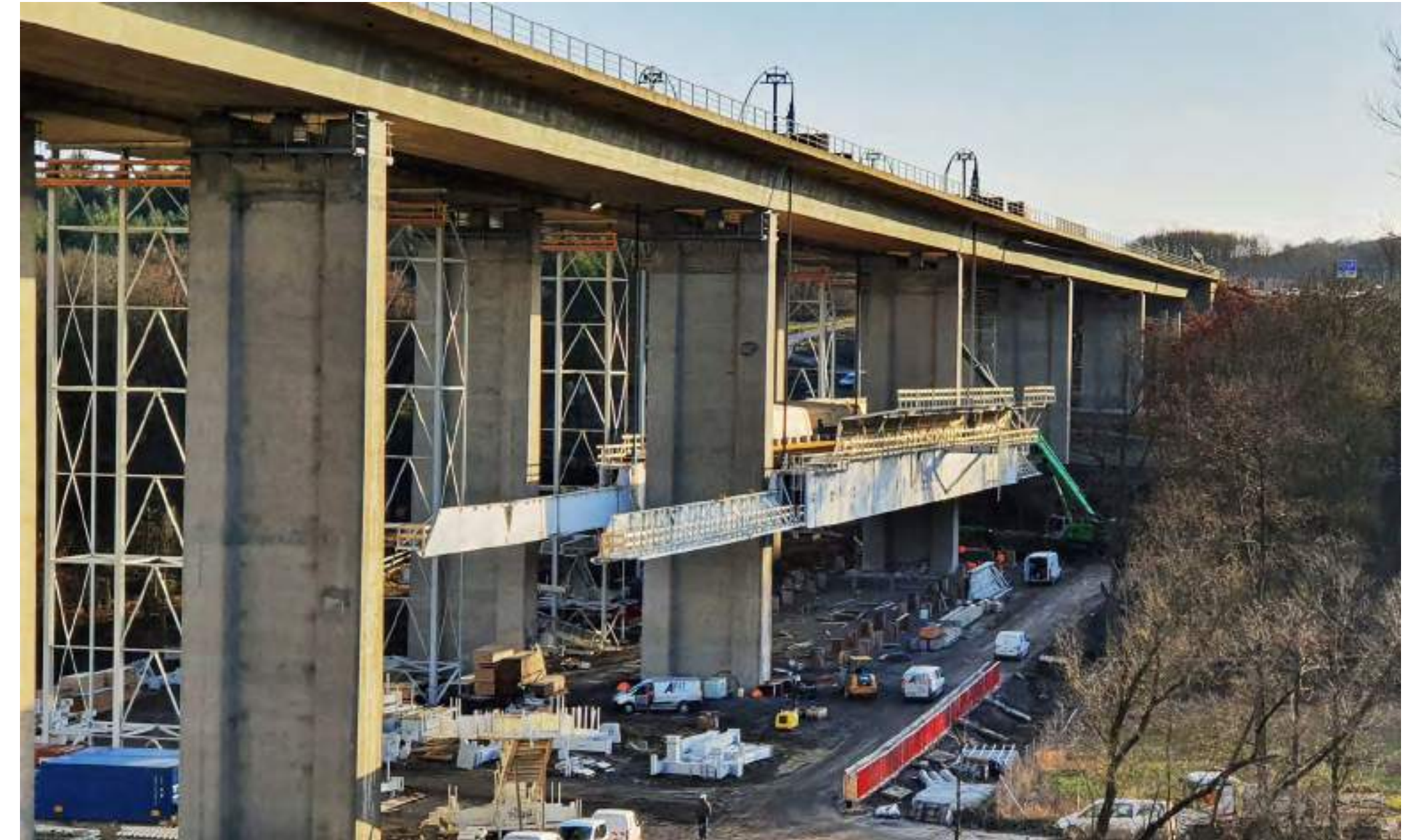
Underslung MSS used at bridge deck demolition– Wertal, Germany
