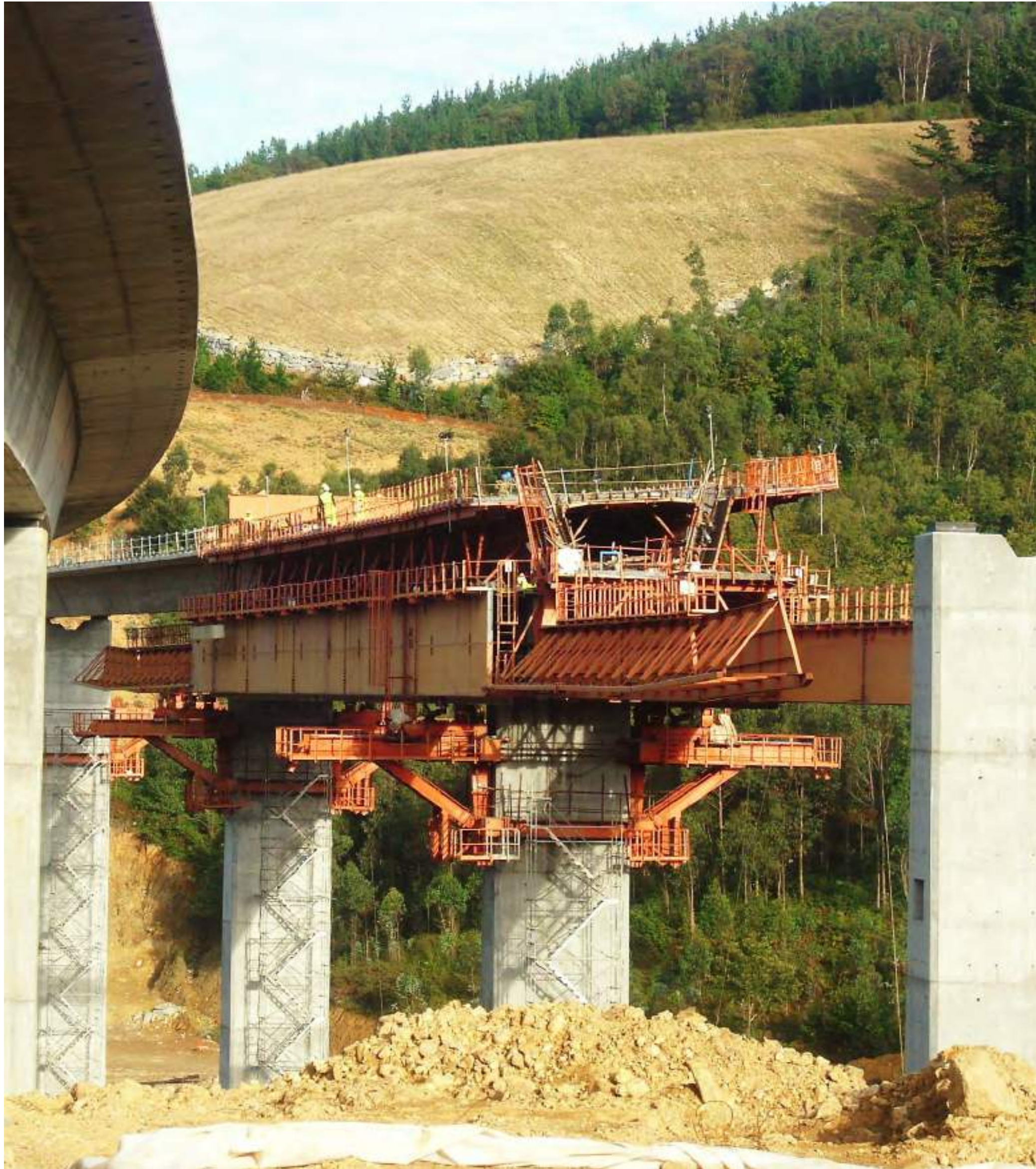
Underslung MSS – Cabirtas, Spain
