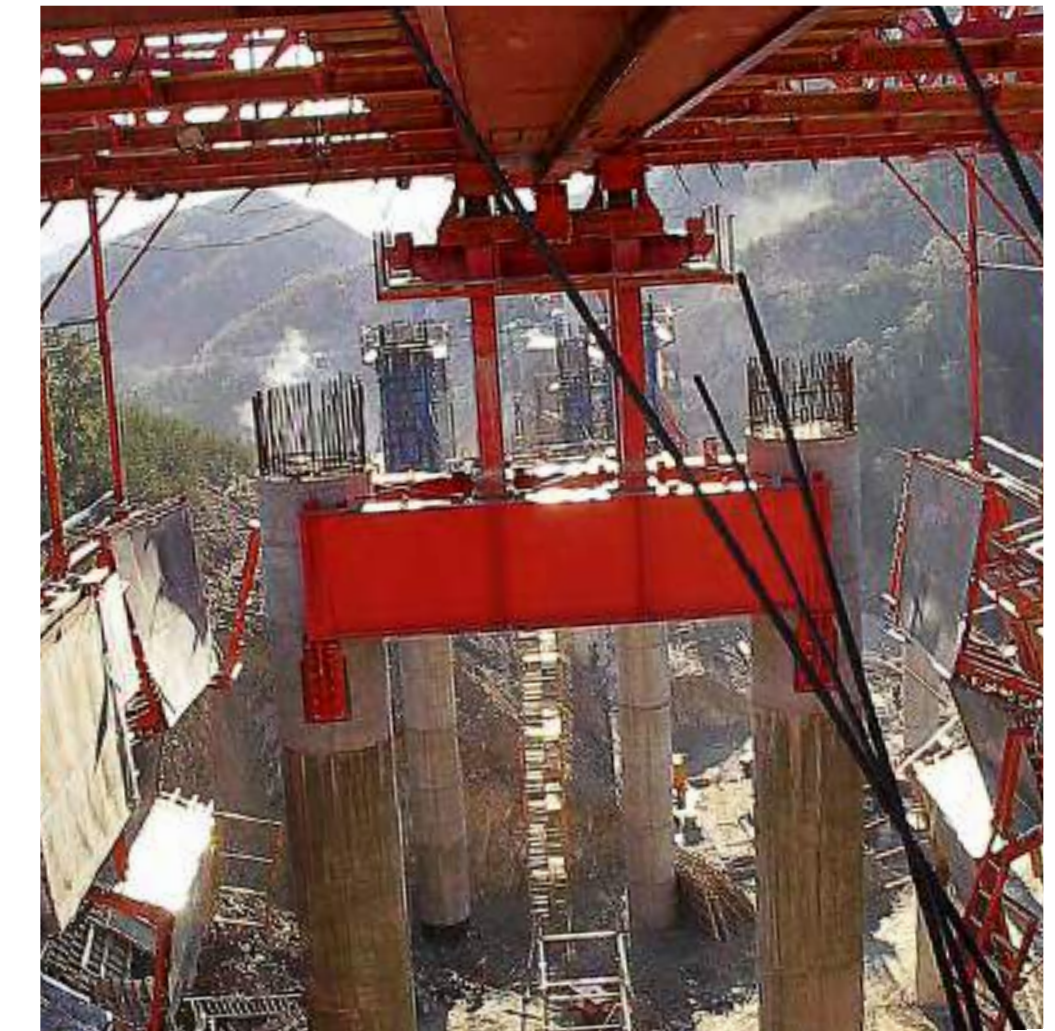
Crossbeam supported on short brackets operating through friction
