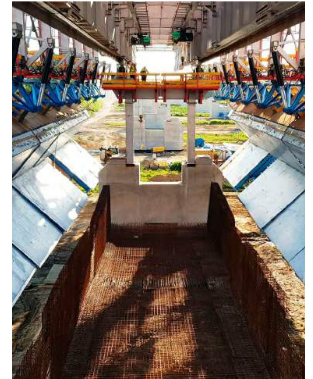
Raising the pre-assembled rebar cage from the ground
