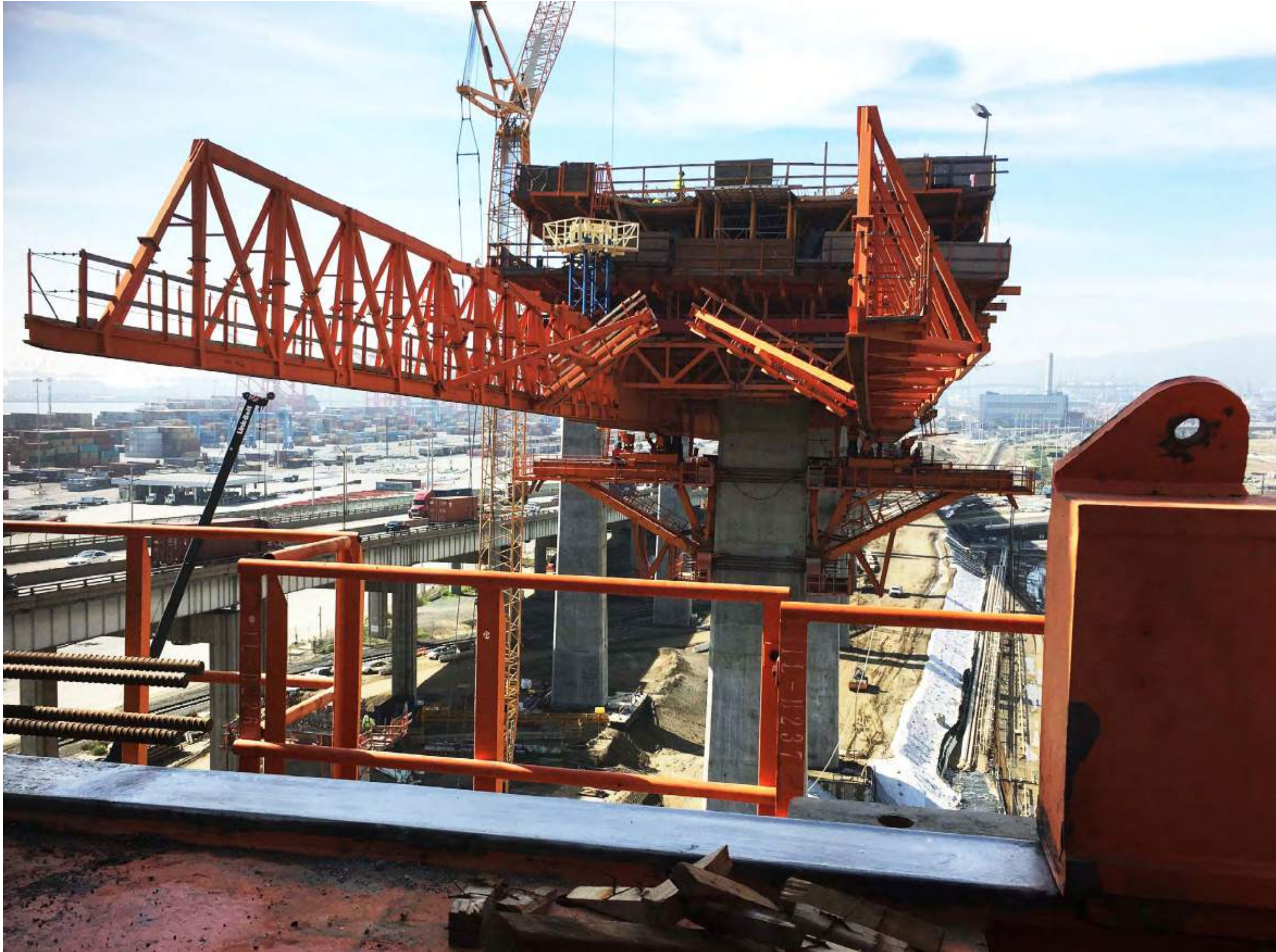
Underslung MSS – Long Beach, USA
