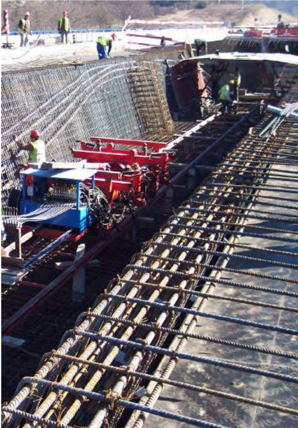
Hydraulic operated transport trolley
