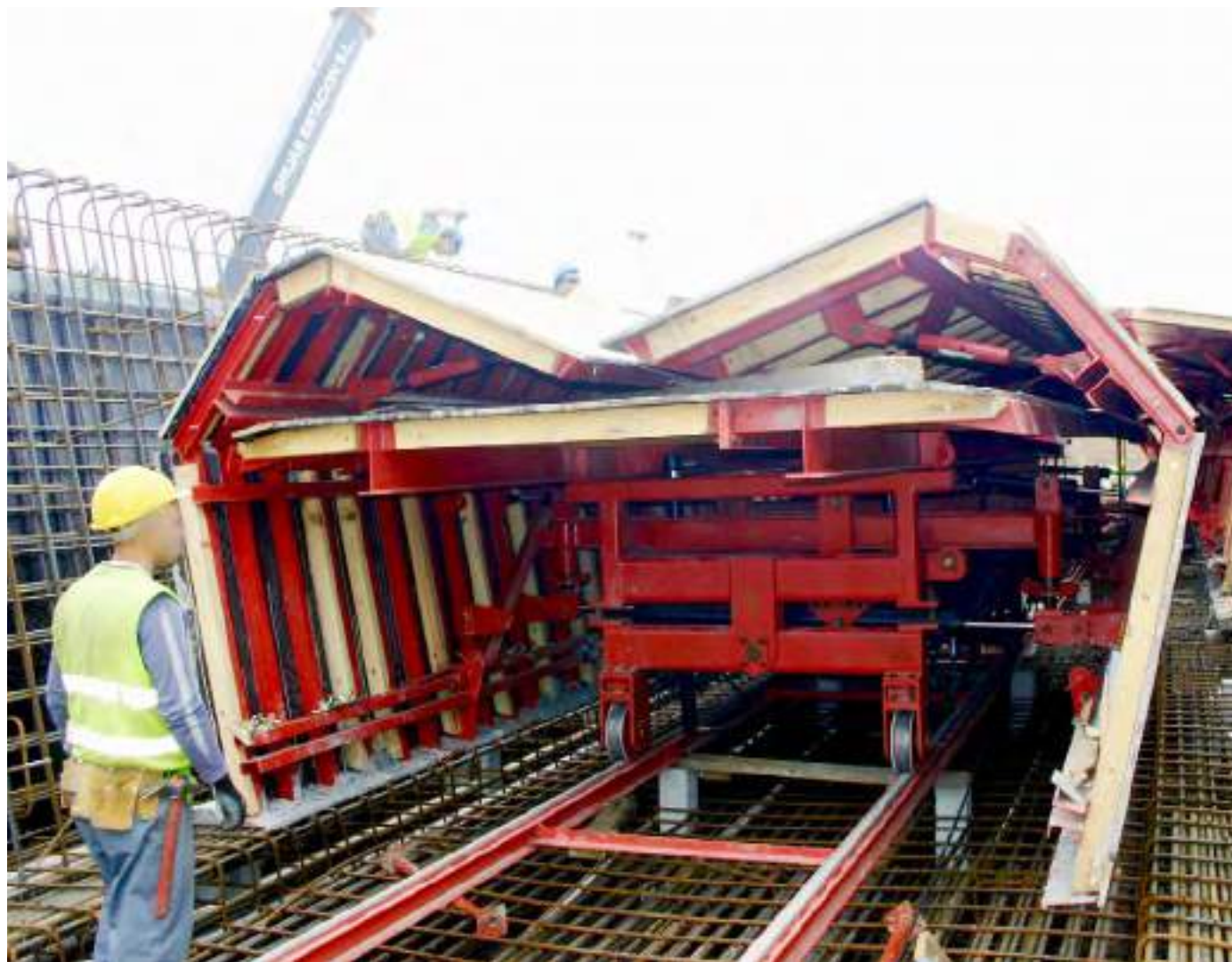
Formwork panel during the transport stage
