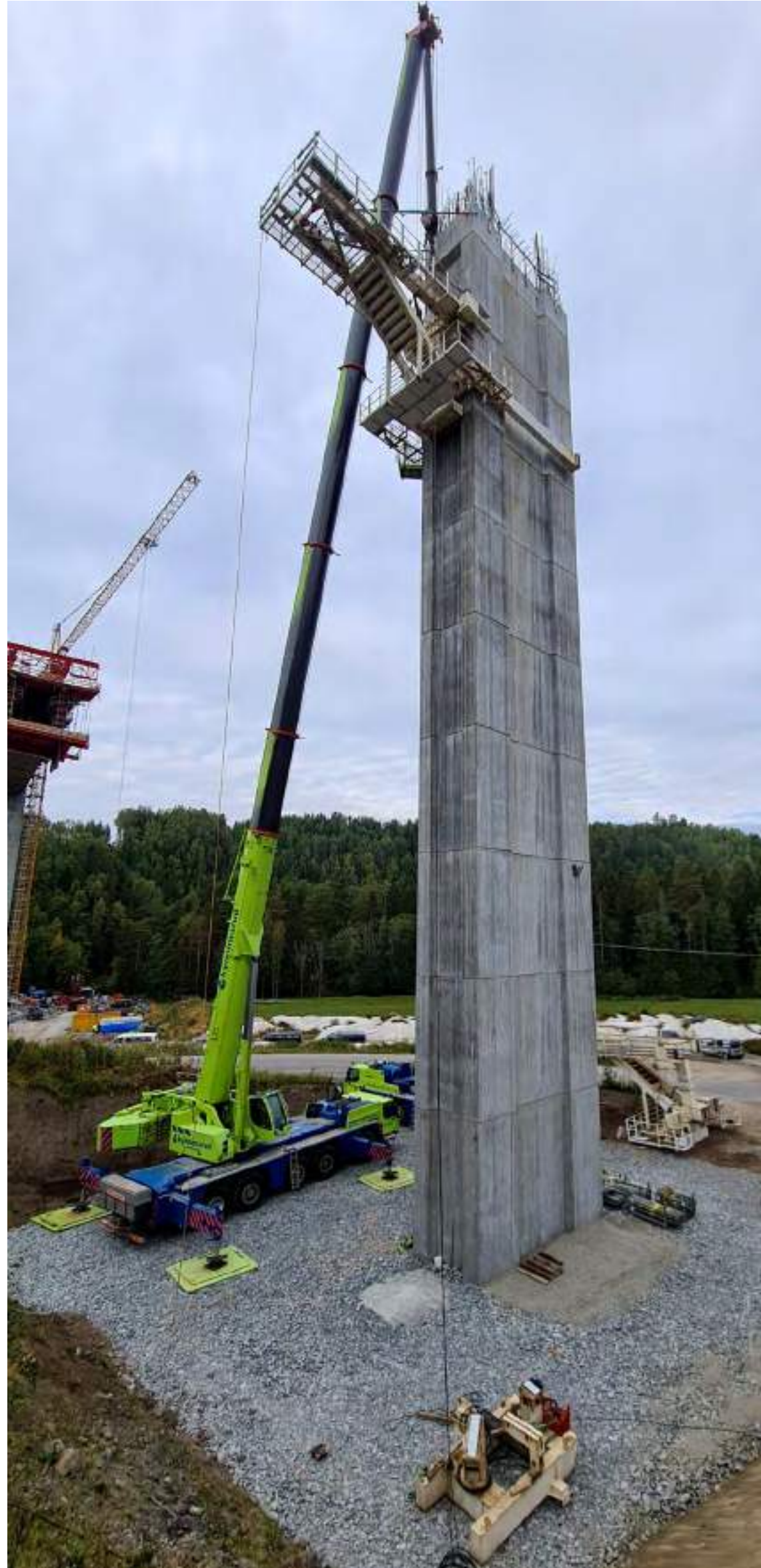
MSS supporting bracket assembling – Randselva, Norway
