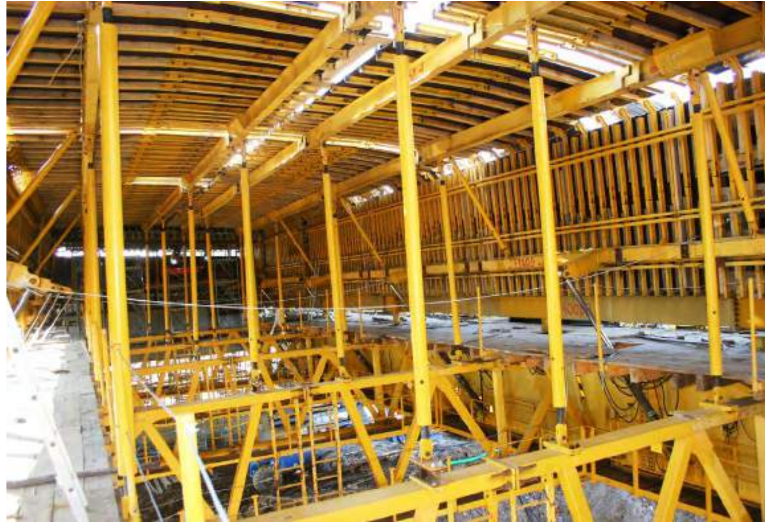
Internal formwork in the closed position
