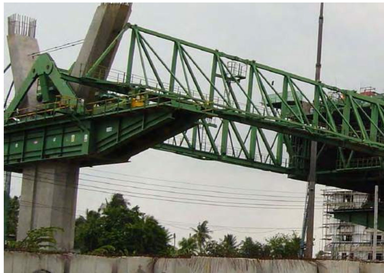
Supporting brackets suspended from the column
