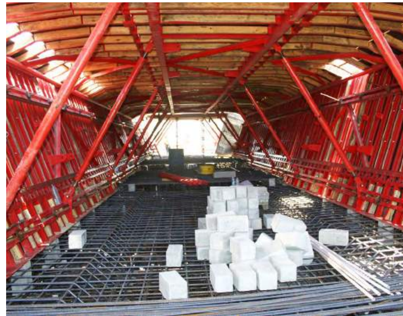
Formwork in the relocation stage on the next span
