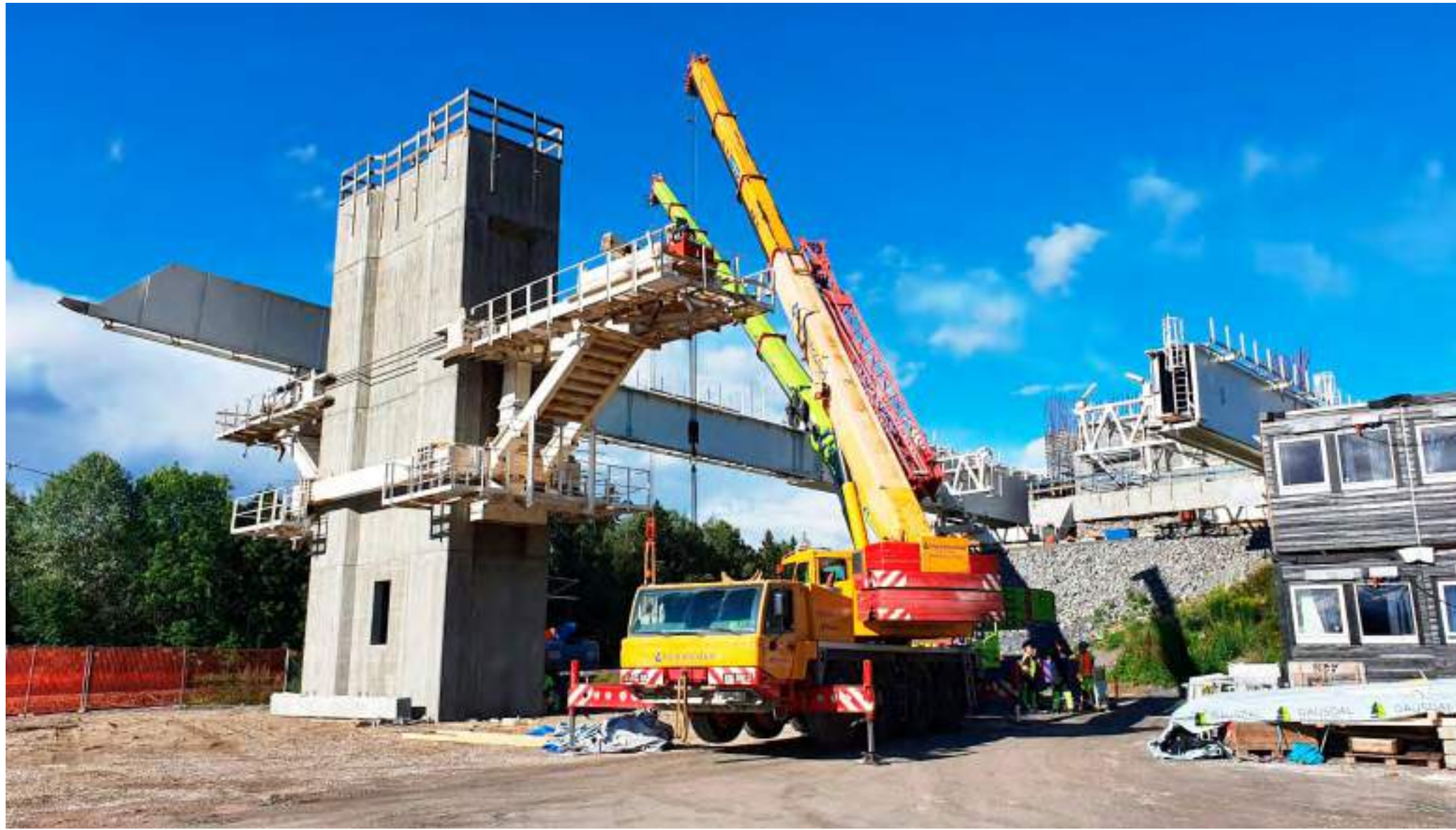
MSS assembling at first span – Randselva, Norway
