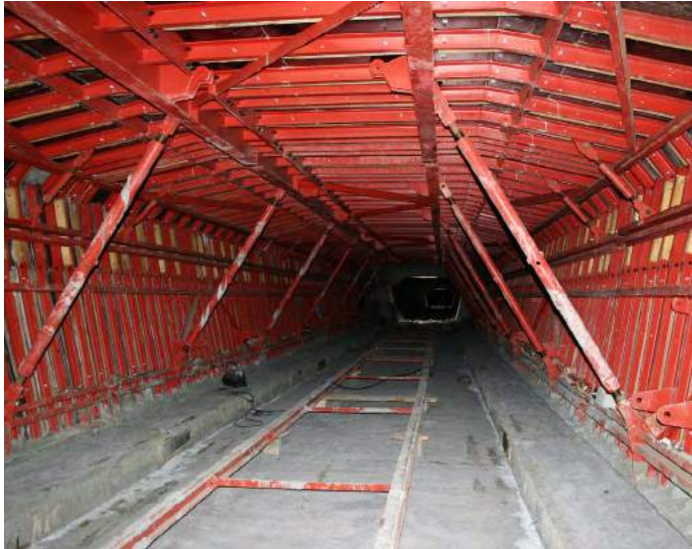
Internal formwork in casting position
