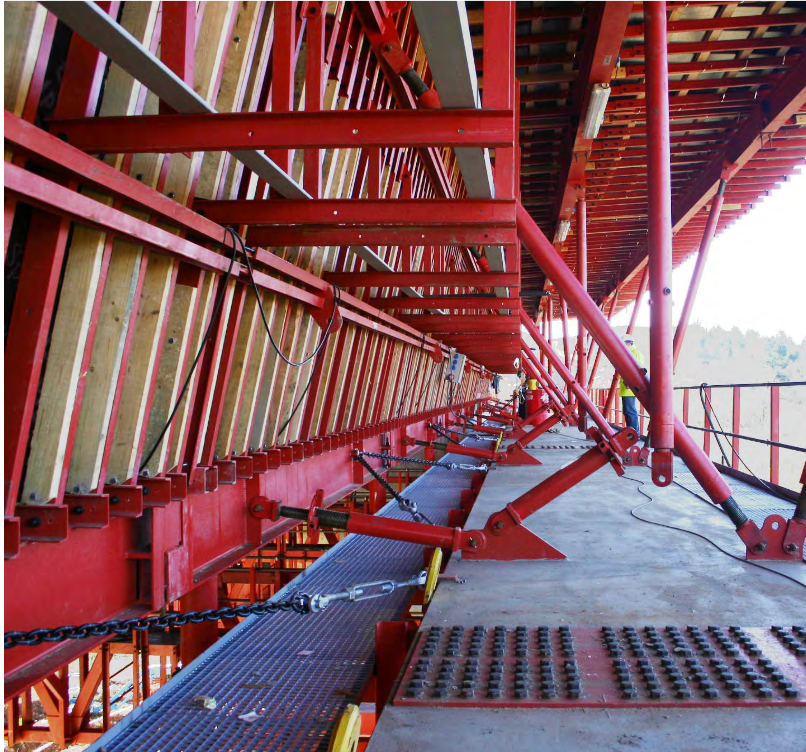
The web and wing external formwork is connected to the bottom formwork by bolts; it is also supported by adjustable struts that help keep the formwork steady and carry out the necessary adjustments.
