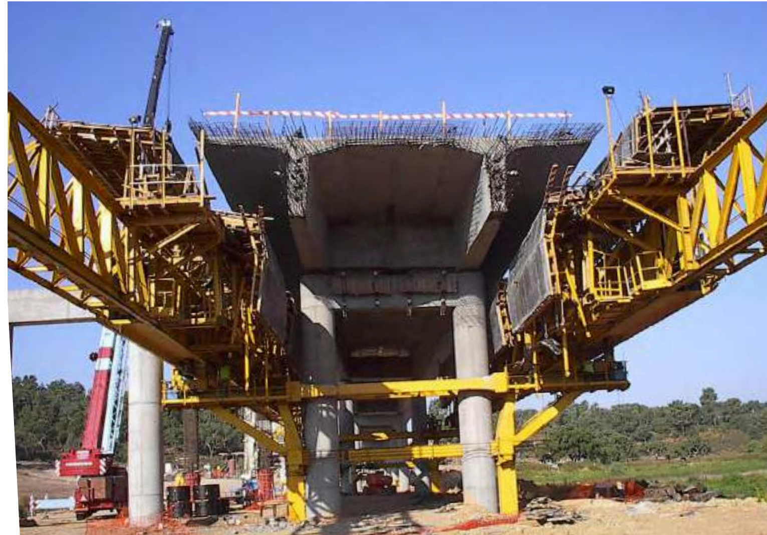
Supporting brackets supported on struts transmitting the reactions to the foundations
