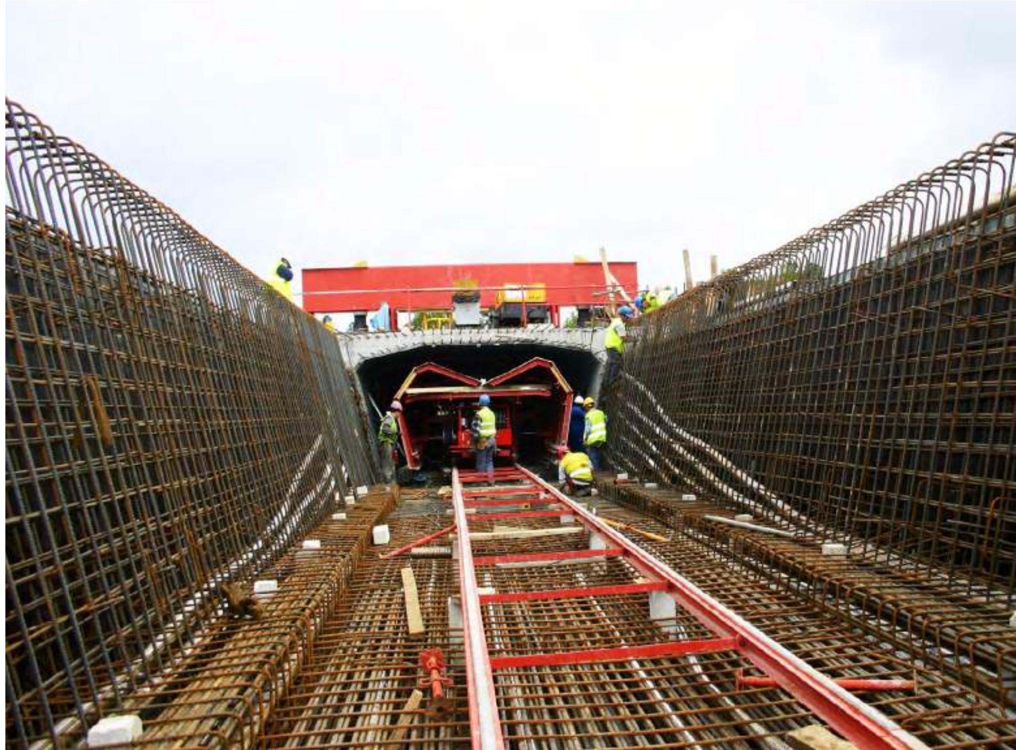
Hydraulic operated transport trolley
