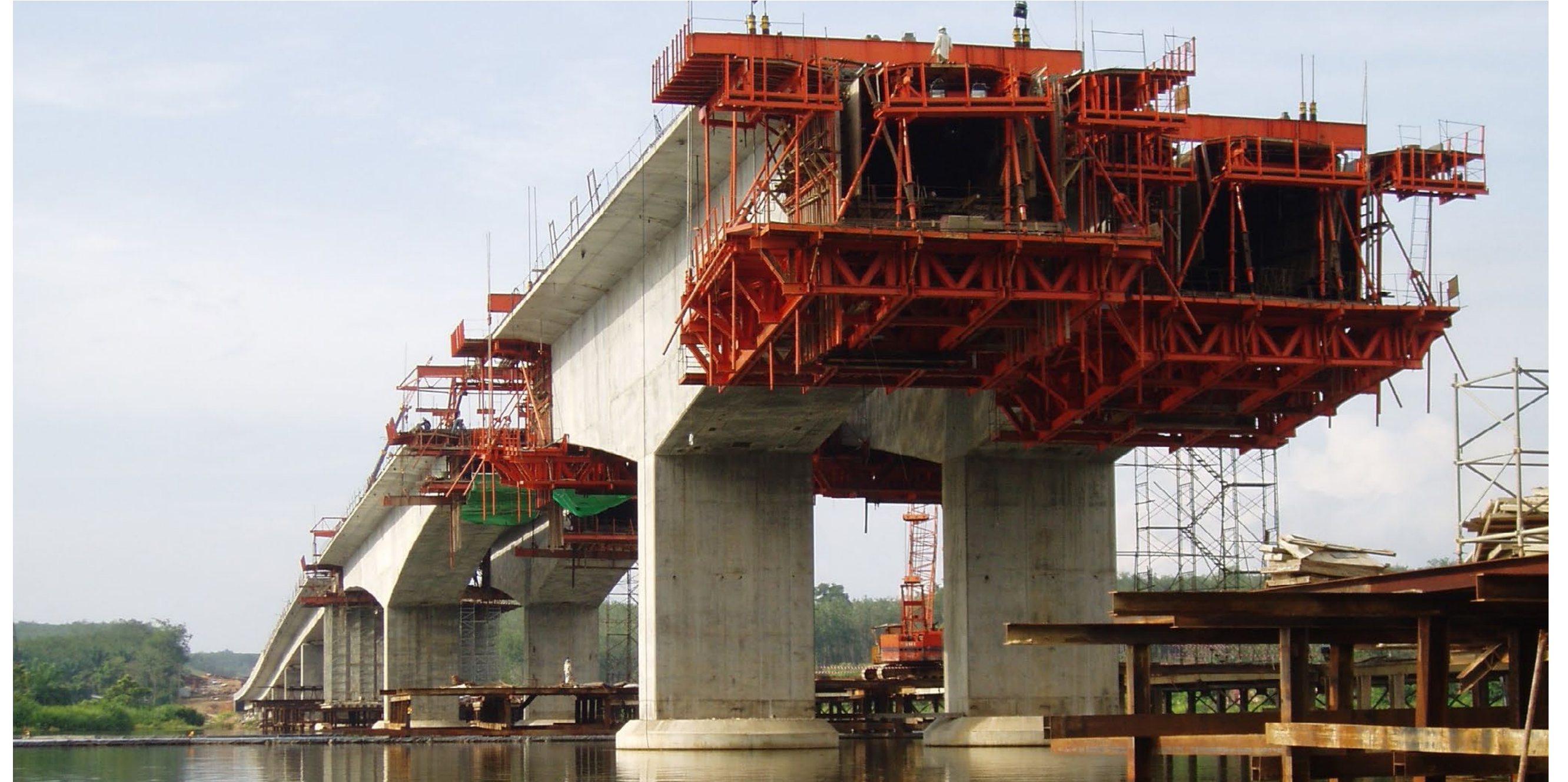
Underslung Form Traveller – Batan Kayan, Malaysia
