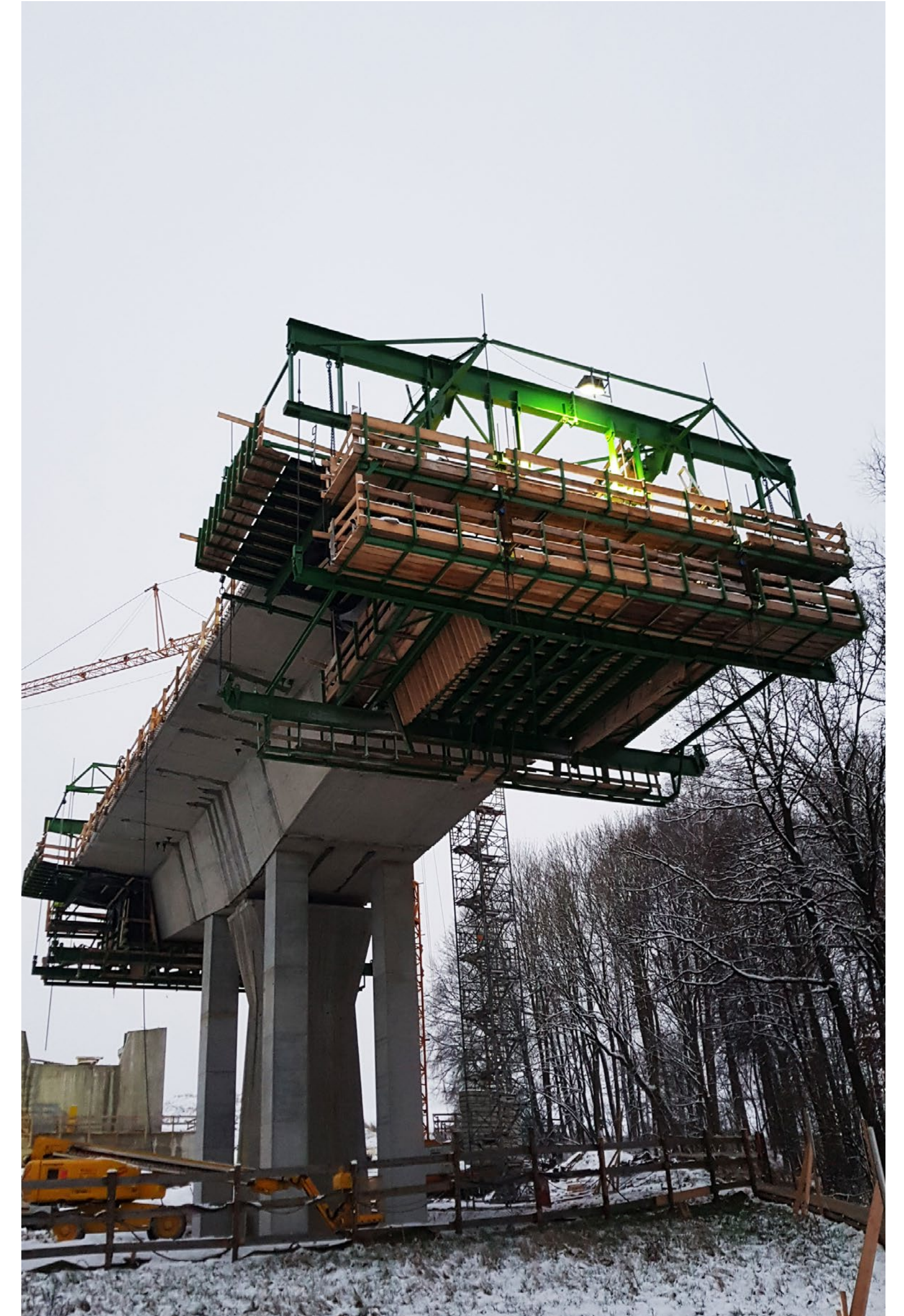
Overhead Form Traveller – Rimbachtal, Germany
