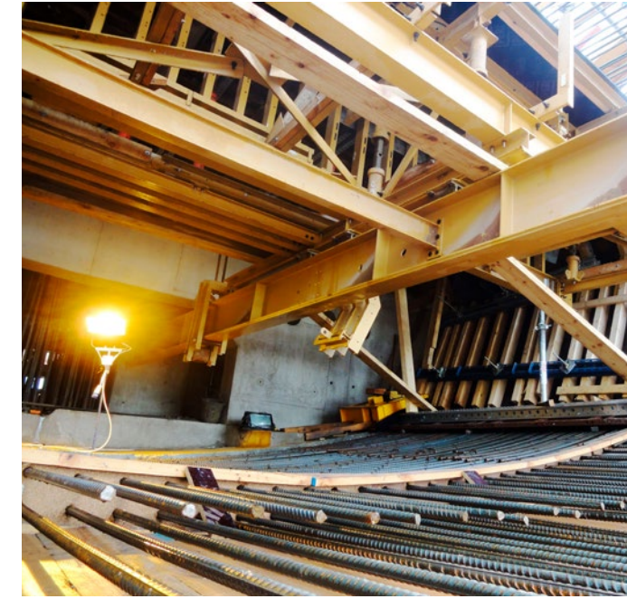
Internal formwork
