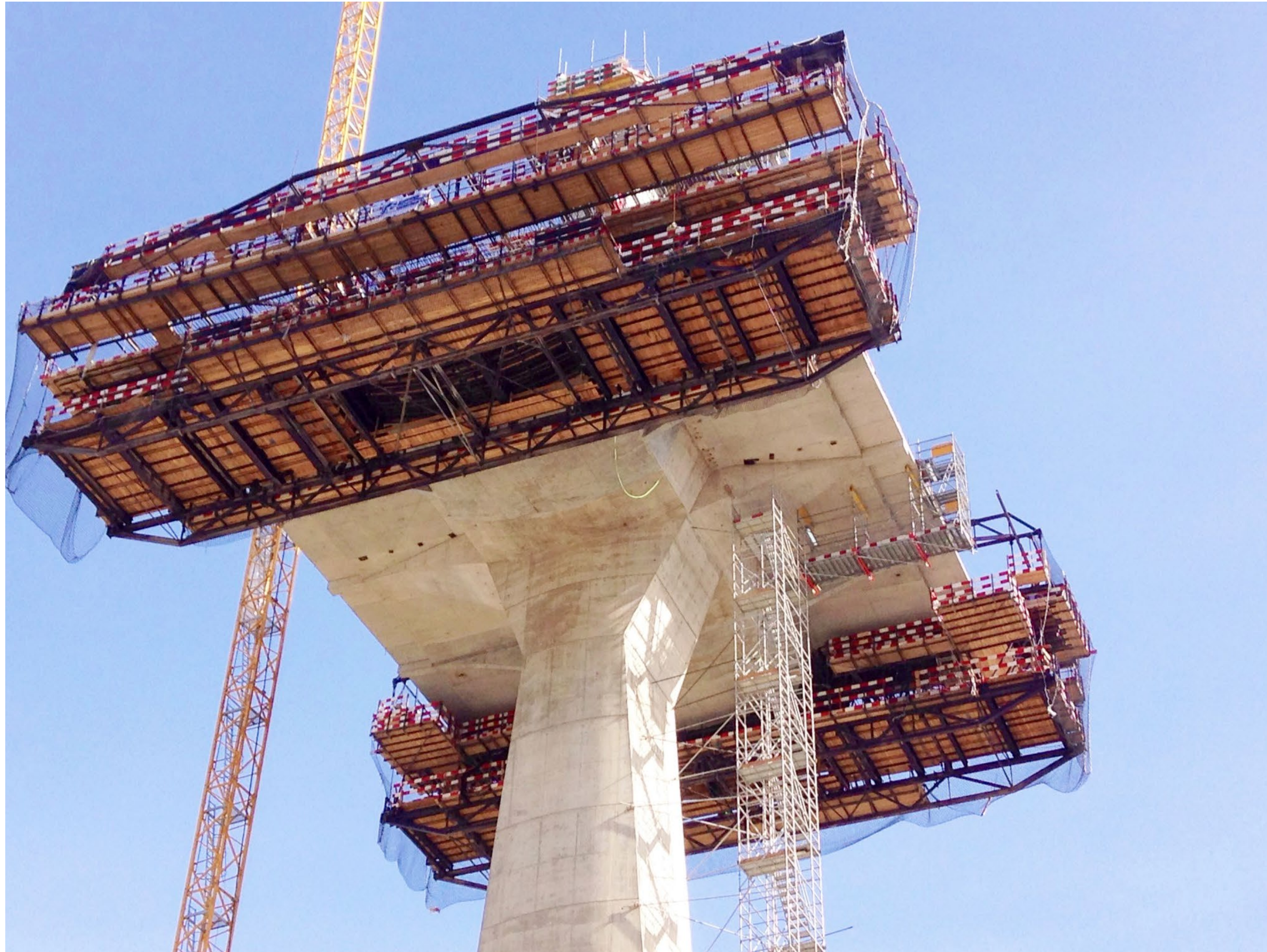
Overhead Form Traveller – Constantine, Algeria
