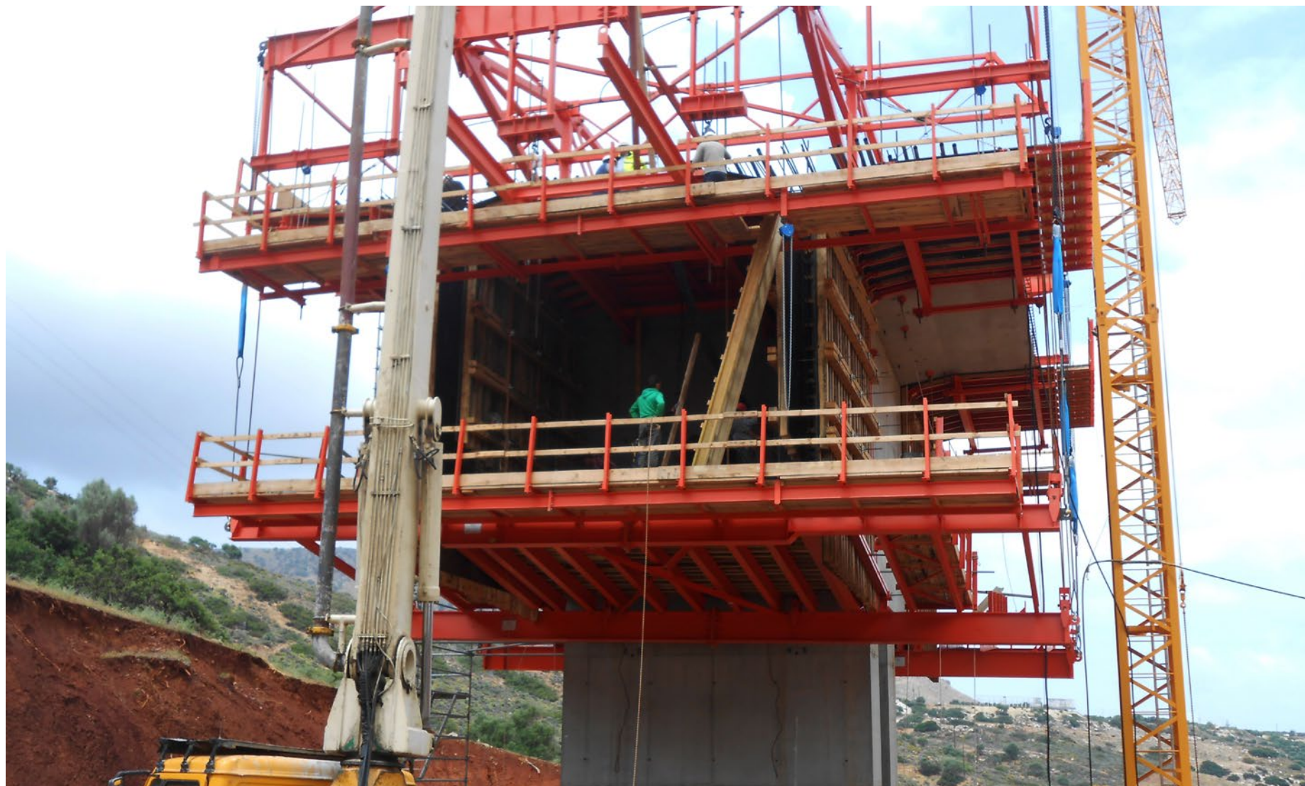
Overhead Form Traveller – Crete, Greece
