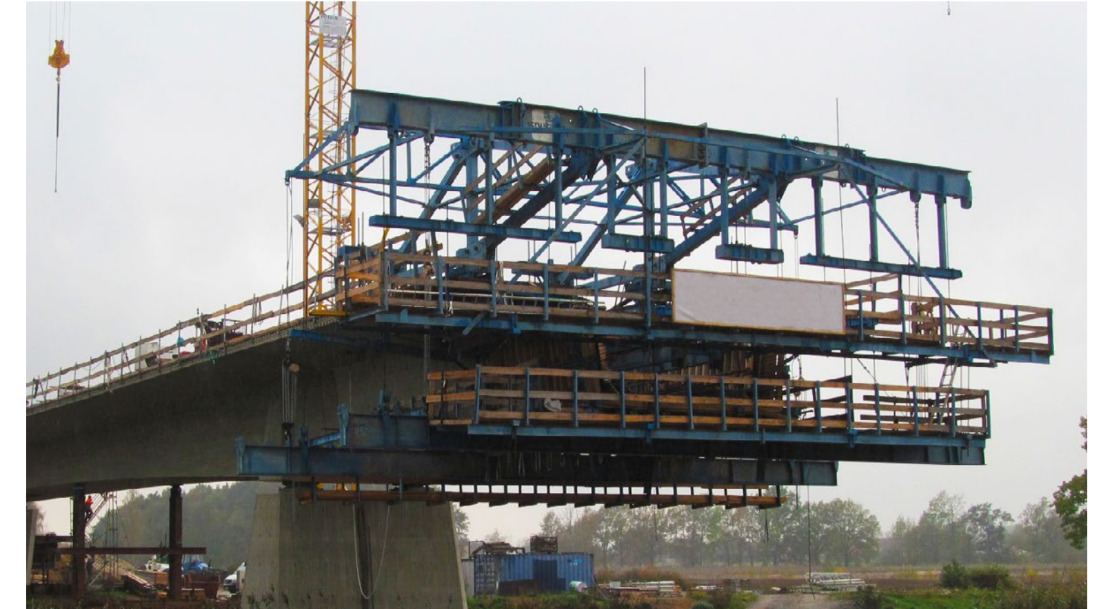
Overhead Form Traveller – Bad Liebenwerda, Germany
