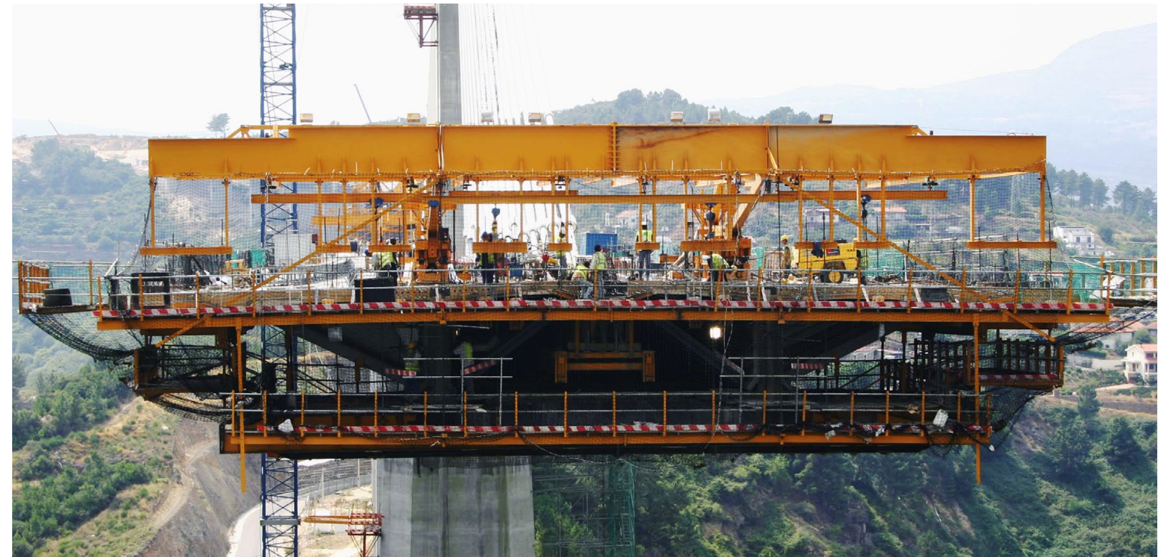
Internal formwork
