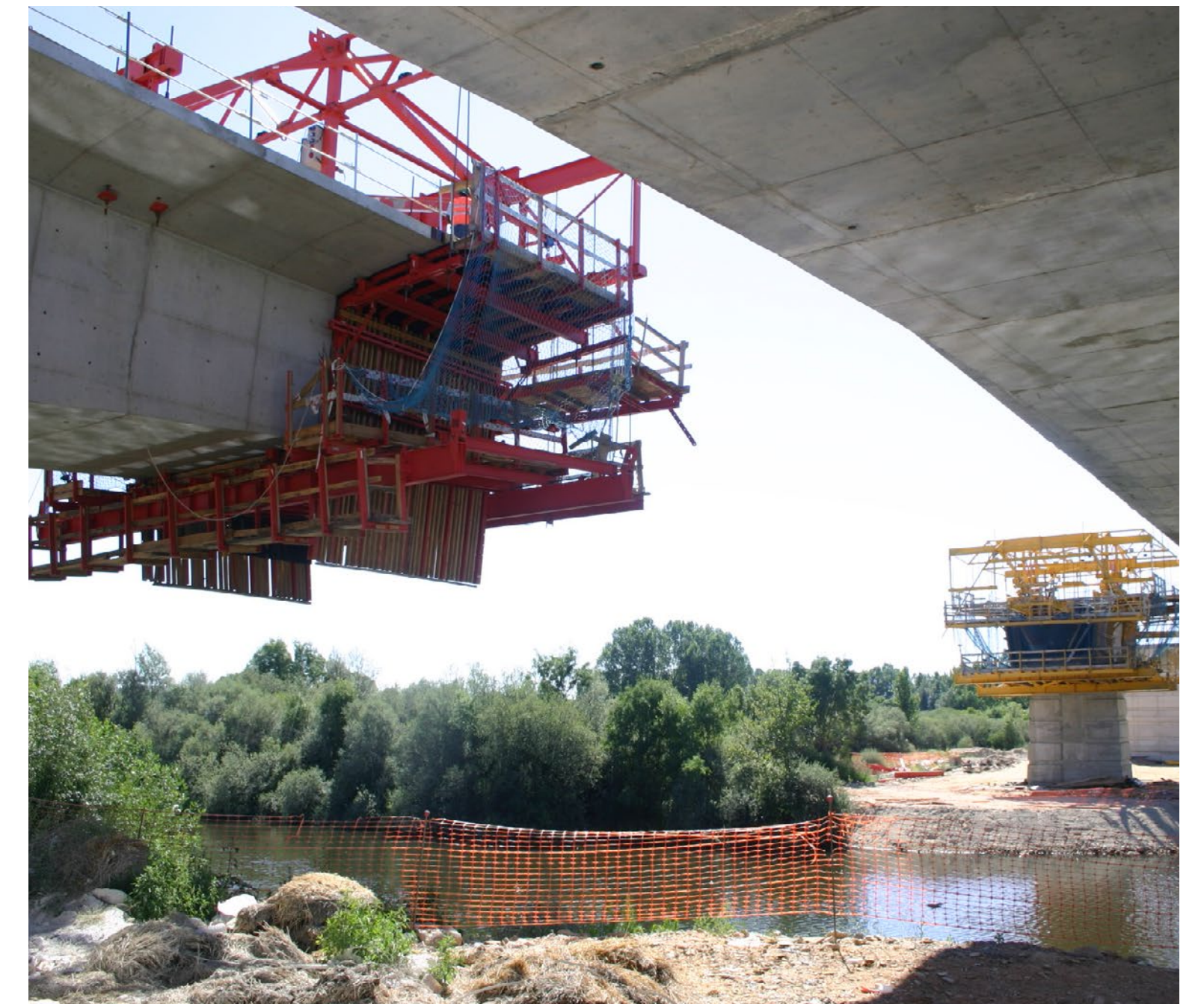
Overhead Form Traveller – Salamanca, Spain
