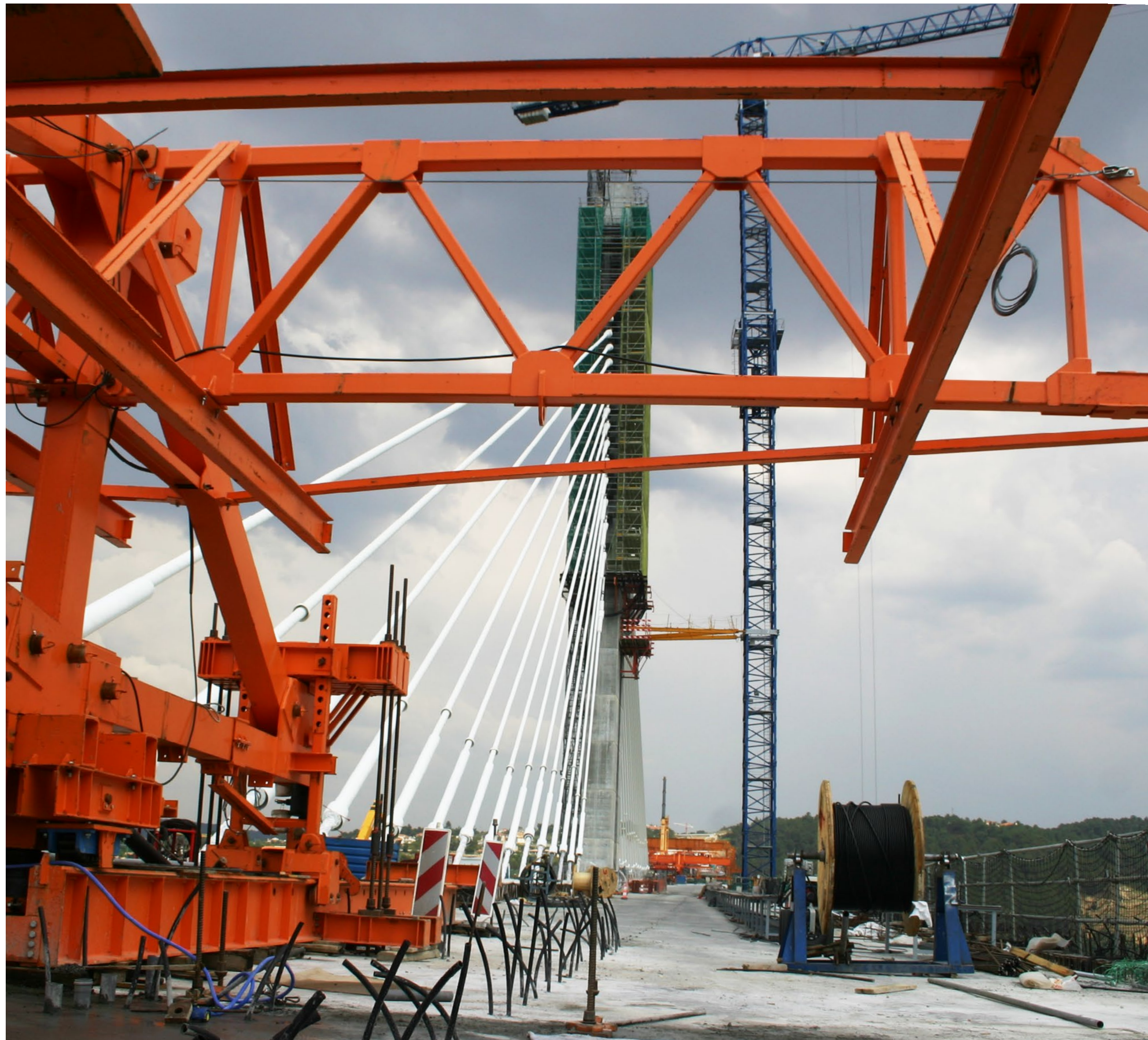
Overhead Form Traveller – Corgo, Portugal
