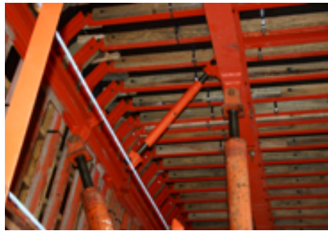
Detail of the formwork plywood fixation
