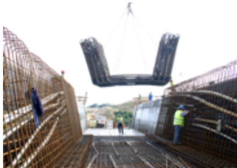
Installing rebar cage deck elements using a mobile crane
