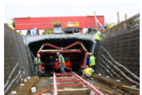
Transport of an internal formwork panel using the rolling wagon hydraulic operated
