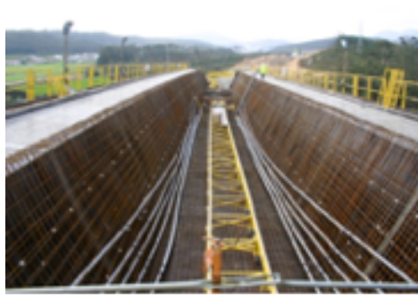
External formwork and rails
