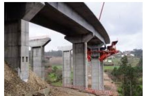
MSS during launching process
