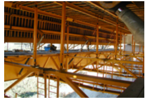
Internal formwork folding cylinders
