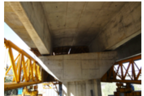
Deck TT cross section without concrete diaphragms
