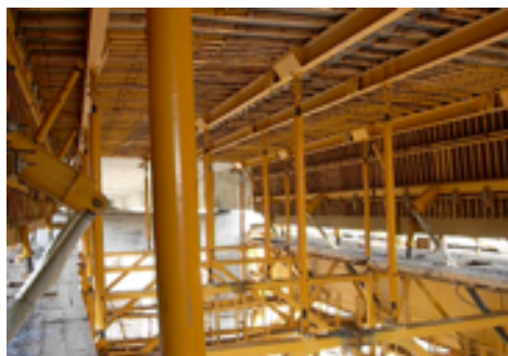
Internal formwork of a TT deck cross section
