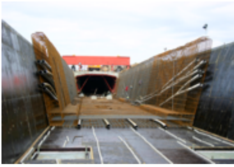
View of the box bottom slab and webs rebar partial installation. Internal formwork still awaiting at previous span.
