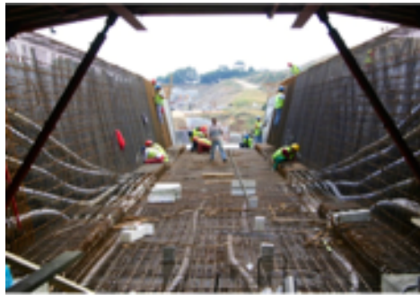
View from the internal formwork front panel towards the new span to be built. Assembling stage of the box bottom slab and web rebar at the new span.
