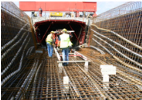
Rails installation on top of precast concrete blocks
