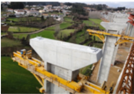
Supporting brackets installed of columns
