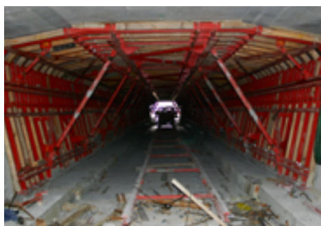
General view of the internal formwork and its transport rolling wagon.
