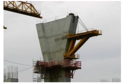
Temporary suspension of the 1st supporting bracket awaiting for the 2nd supporting bracket of the pair
