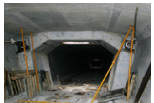
Detail of the diaphragm opening above column alignment to permit to pass with the internal formwork panel and its transport rolling wagon
