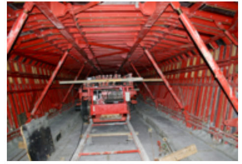
Internal formwork rolling wagon starting the rails transport
