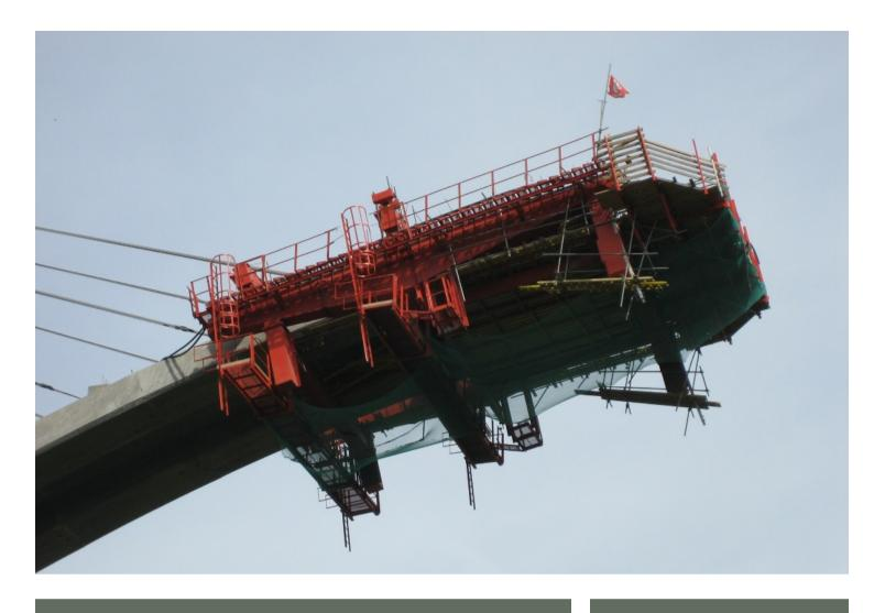
The formwork surfaces in contact with the concrete can be wood, film faced plywood, metal sheet or plastic plate, depending on the number of reuses envisaged and the concrete architectural requirements.
